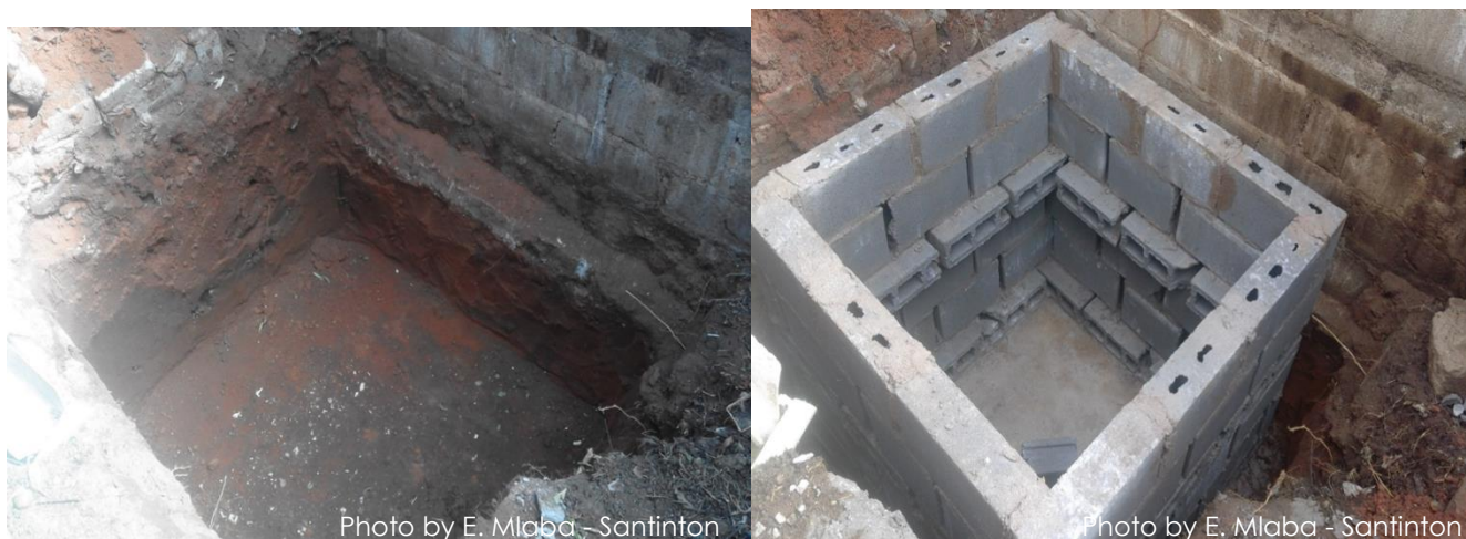
From left: leach pit hole before and after the insertion of blocks
