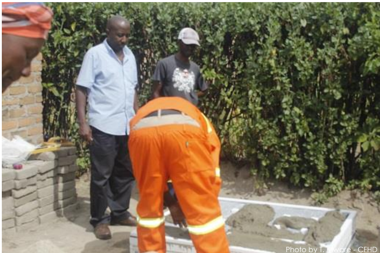
Casting of sheets that were used in the construction of leach pit
