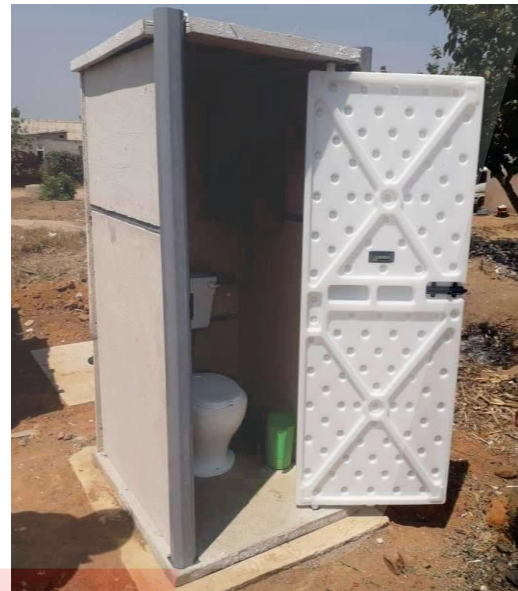
An installed easy-flush toilet in Epworth, Ward 3
